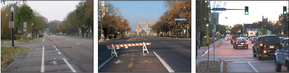
Fig. 2. Examples of left side losers (the bicycle lane ends in all shown examples).
